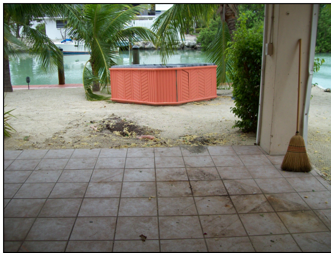
Figure 17. Hot tub blown out from underneath house at 393 Palm Drive.
