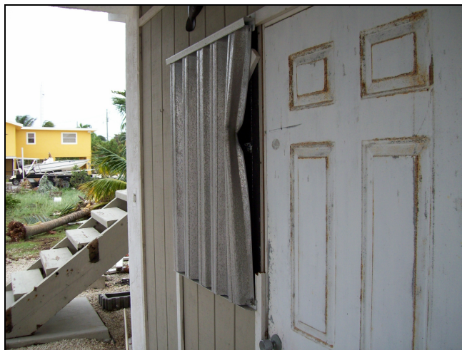
Figure 5. Damage to back porch of 153 Iroquois Dr.
