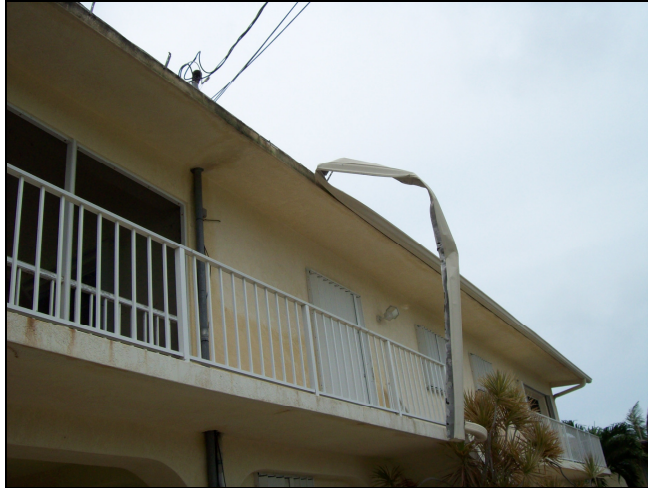
Figure 10. Front view of house at 100 Willow Lane.
