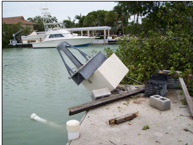
Figure 26. Close up view of rightmost davit at home at 210 Buttonwood Lane. Note top rail of fence on seawall as well as cinder blocks blown from right side of picture. Also note broken seawall bumper in canal.
