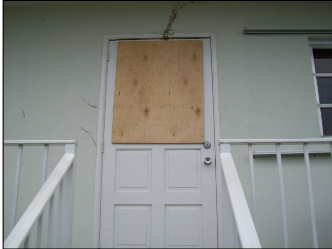
Figure 18. Home at 399 Palm Drive with front door damage. Door faces east.
