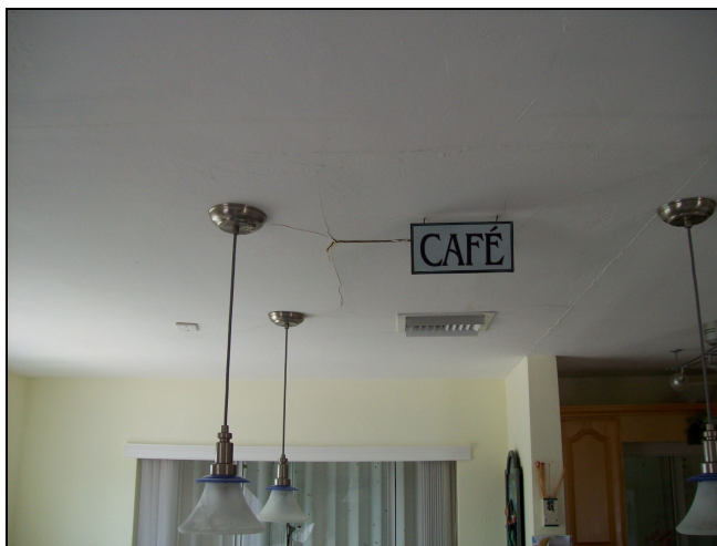
Figure 16. Dining room ceiling of house at 393 Palm Drive whose roof was damaged. Note the window in the background through which a tree limb came through. This view is looking approximately southeast.
