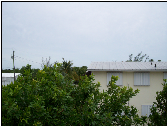
Figure 20. Looking back to east southeast from home at 399 Palm Drive with door damage.
