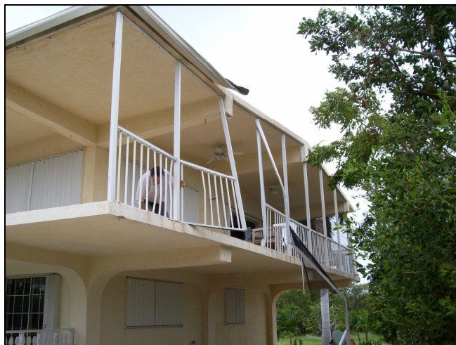
Figure 9. Porch Damage at house at 100 Willow Lane.
