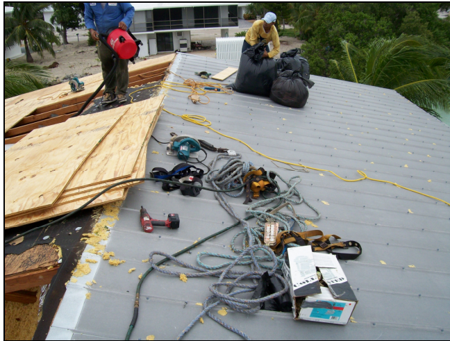
Figure 15. Roof damage to house on Palm Dr. View is looking approximately south.
