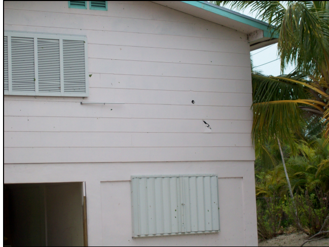
Figure 12. House on Palm Dr with siding damage.
