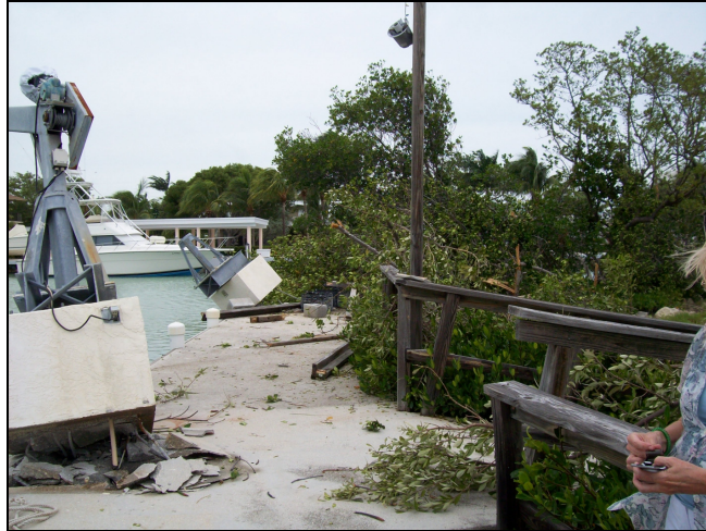
Figure 25. View looking north northeast from backyard of 210 Buttonwood Lane. Note apparent travel of tiki hut would have been from right to left and just beyond electric pole in center of photo. Rightmost davit in background.
