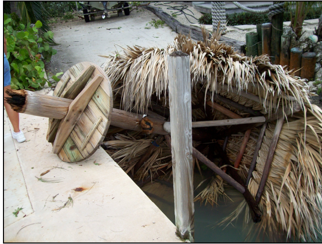
Figure 23. Tiki hut snapped and blown into adjacent boat ramp.
