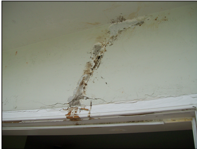
Figure 19. Close up view of damage above door in Fig. 18.
