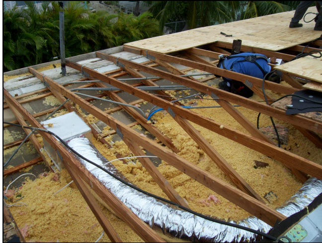
Figure 14. Roof damage at house on Palm Dr.
