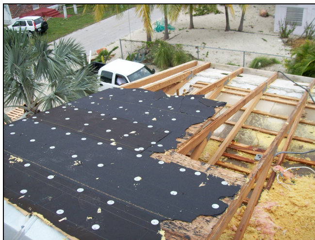
Figure 13. Roof damage at house at 393 Palm Dr. View is looking east southeast.
