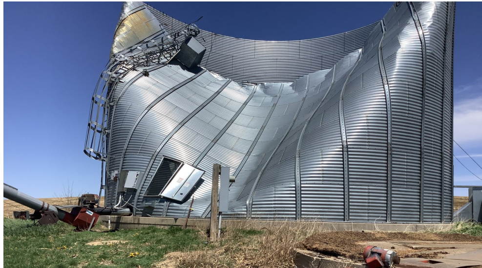
Figure 2. Grain bin which lost its cap and was pushed in by the intense winds on May 12th
