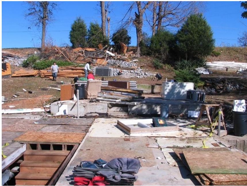
The image to the left shows damage caused by this EF-1 tornado that struck just southeast of Bowling Green.
