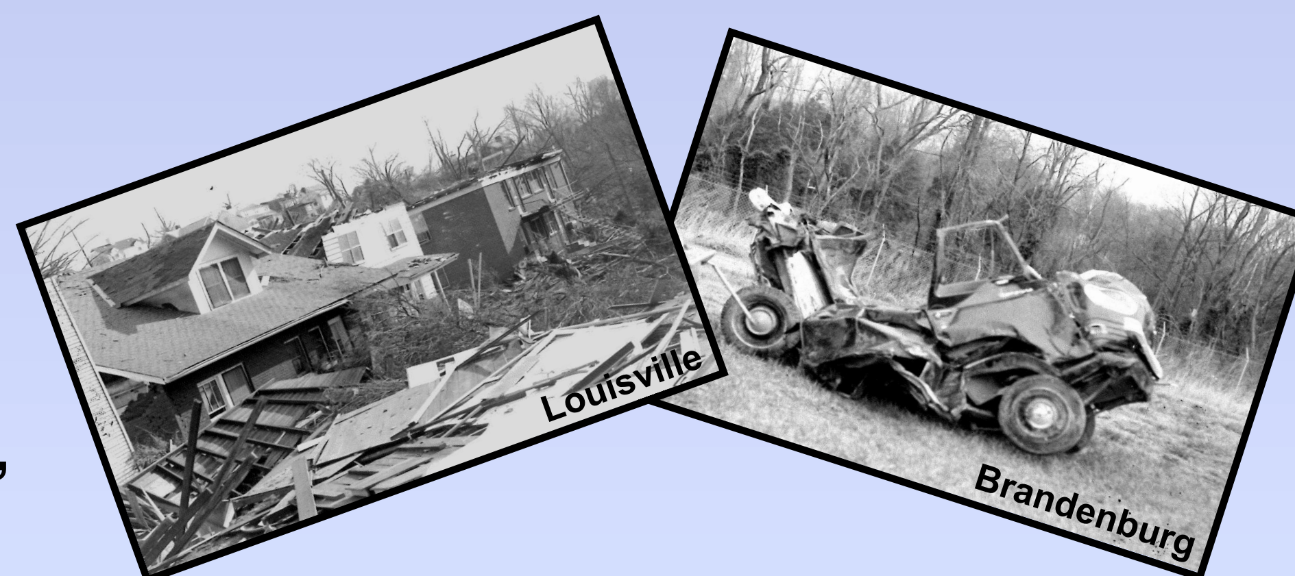
On April 3, 1974 a tornado touched down just half a mile from the weather office and grew to F4 strength as it plowed through northeastern Louisville and into Oldham County. The weather office was battered by 84 mph winds, knocking over the meteorological instruments that were on the office's roof.
