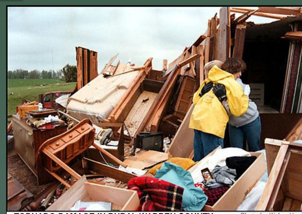
TORNADO DAMAGE IN RURAL WARREN COUNTY
