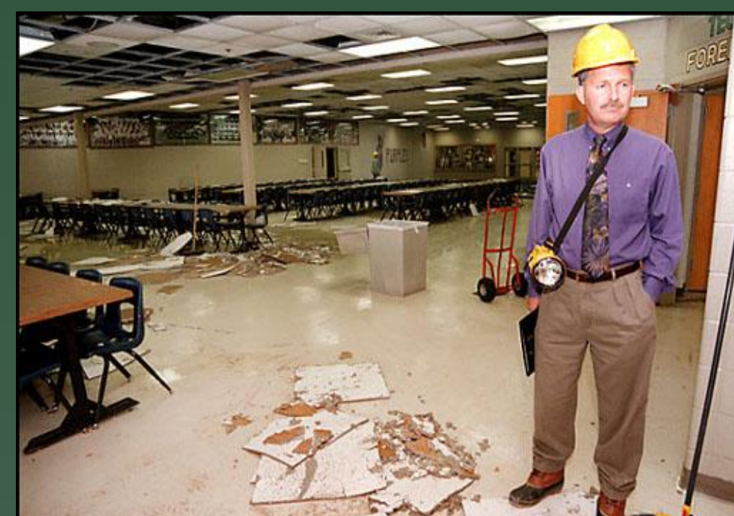
BOWLING GREEN HIGH SCHOOL HAIL/WATER DAMAGE
