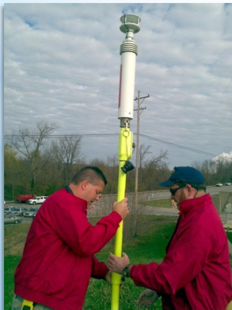
Toby TenHarmsel and Joe Sullivan install a temporary weather station.
