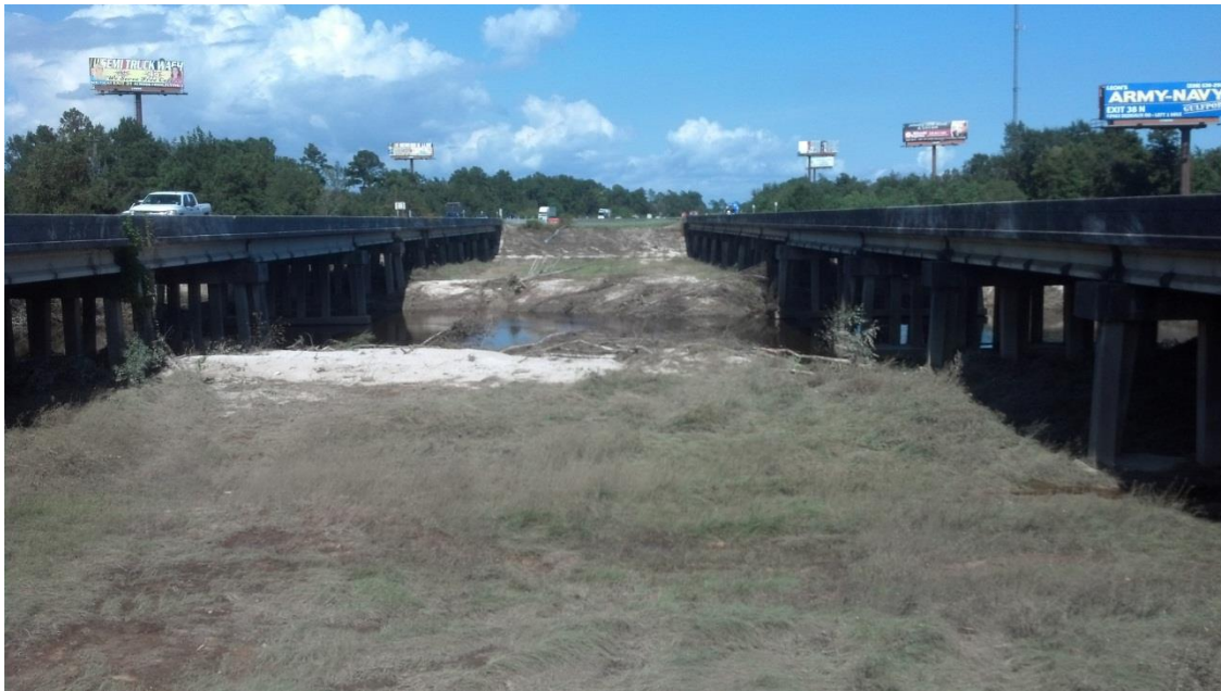
419 420 Figure 15. Downstream view from Cable Bridge Rd. Widespread damage to trees and brush 421 were noted. 422
