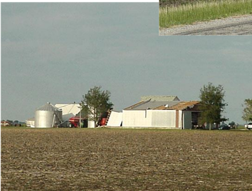
Second machine shed damaged by the tornado. The nearby farm home also sustained roof and window damage. Viewing northeast.
