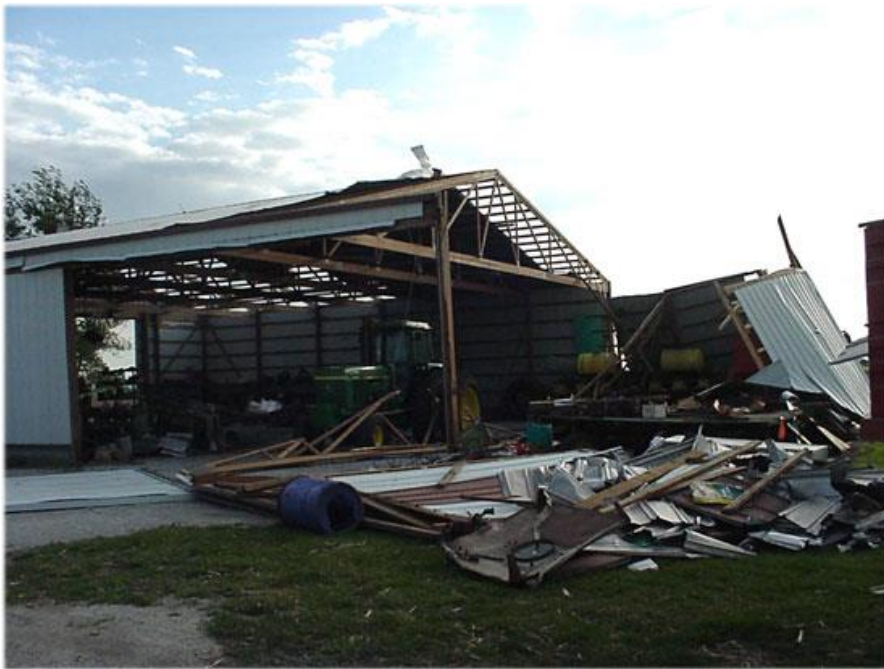
Northern part of the machine shed. Debris from the machine shed was tossed several hundred feet to the southeast. Viewing southwest.
