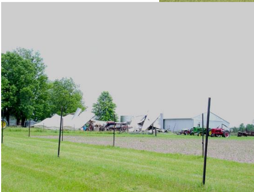
A machine shed on Hastings Cemetery Road was destroyed on this farm by the first tornado. Debris from the machine shed was tossed to the east-southeast. Viewing east-southeast. Much of the damage associated with the three weak tornadoes was tree damage.
