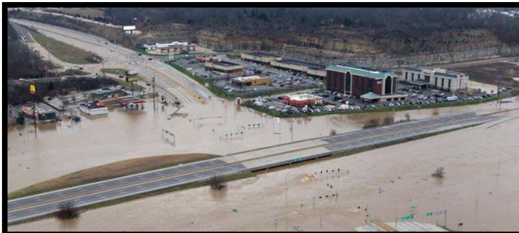
Meramec River Flooding in Valley Park, Missouri Photo Courtesy of St. Louis Post Dispatch
