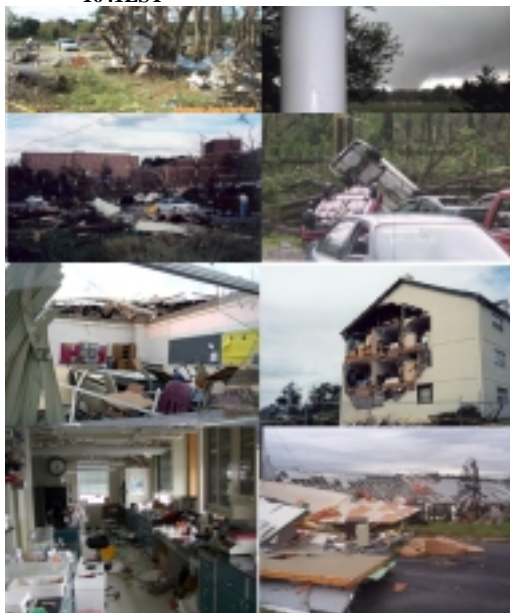
Damage from tornado that tracked across northern Prince George's and Eastern Howard Counties: Top row left: Remnants of 10 Maryland Fire and Rescue Training Institute trailers at the University of Maryland (photo by Kay Graham, PG Co. OEP); right: The large wedge-shaped tornado as it crossed through the western portion of the University of Maryland (from terpidots.com website); 2nd row left: Another picture of what remains of the Fire and Rescue Institute trailers with a dorm in the background (photo by Kay Graham); right: Several flipped cars in a student parking lot near destroyed trailers (from terpidots.com website); 3rd row left: Roof was removed from three classrooms at Laurel High School (Copyright 2001, The Baltimore Sun, Photo by Kenneth Lam); right: Side of a brick apartment building in Beltsville was blown out (photo by Kay Graham); Bottom row left: Damage to experiments inside a building at the USDA Beltsville Agricultural Research Center (BARC) (photo from USDA BARC); right: Roof debris and one of many destroyed greenhouses at BARC (photo from USDA BARC).
