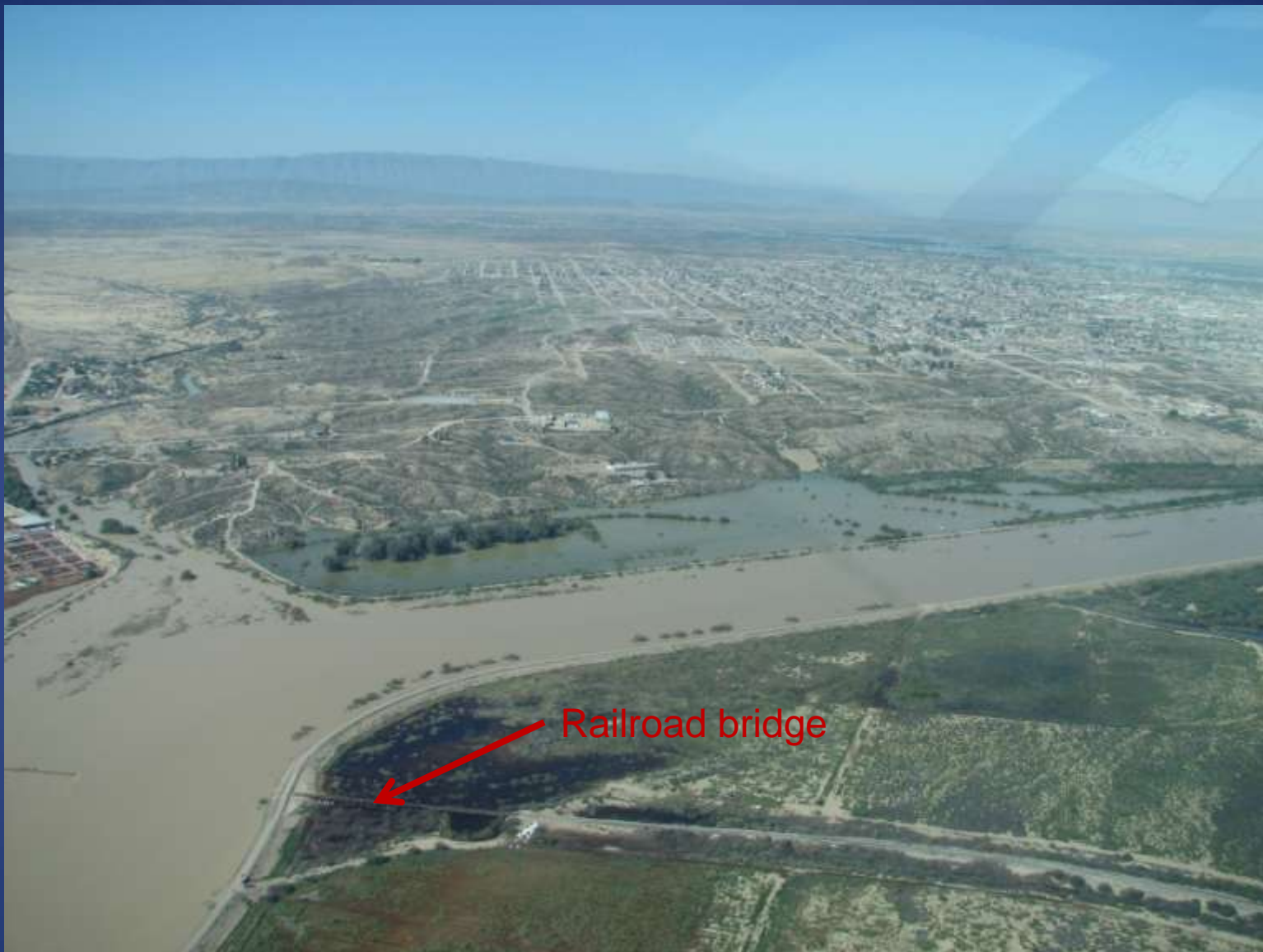
Rio Grande about 1.6 miles downstream of International Bridge (Railroad bridge in lower left of picture)
