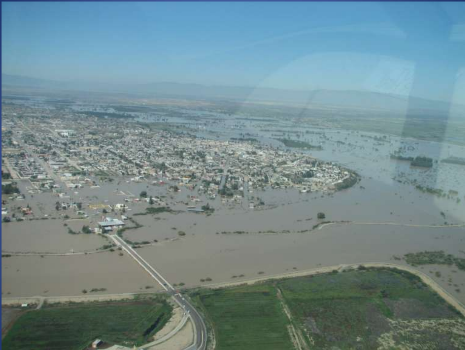
Looking upstream from International Bridge (Ojinaga, MX in background). RG_09_20_08 053
