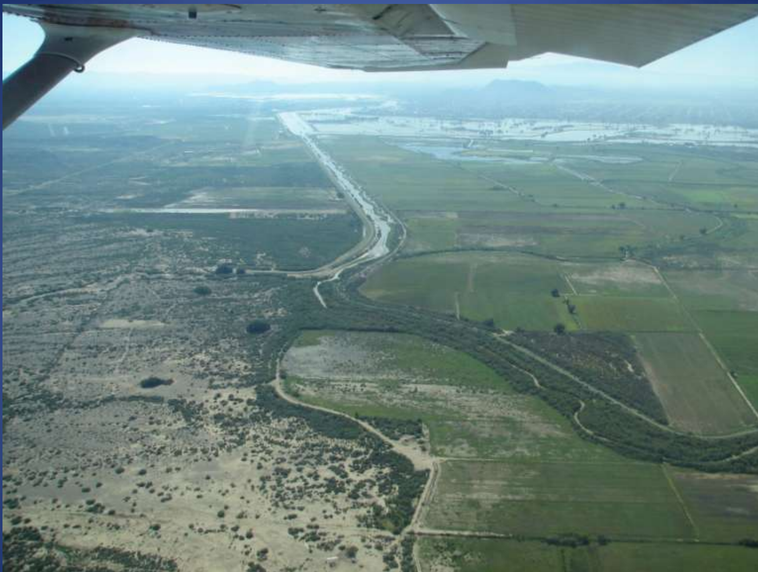
Rio Grande upstream of Presidio - looking downstream at start of levees RG_09_20_08 035
