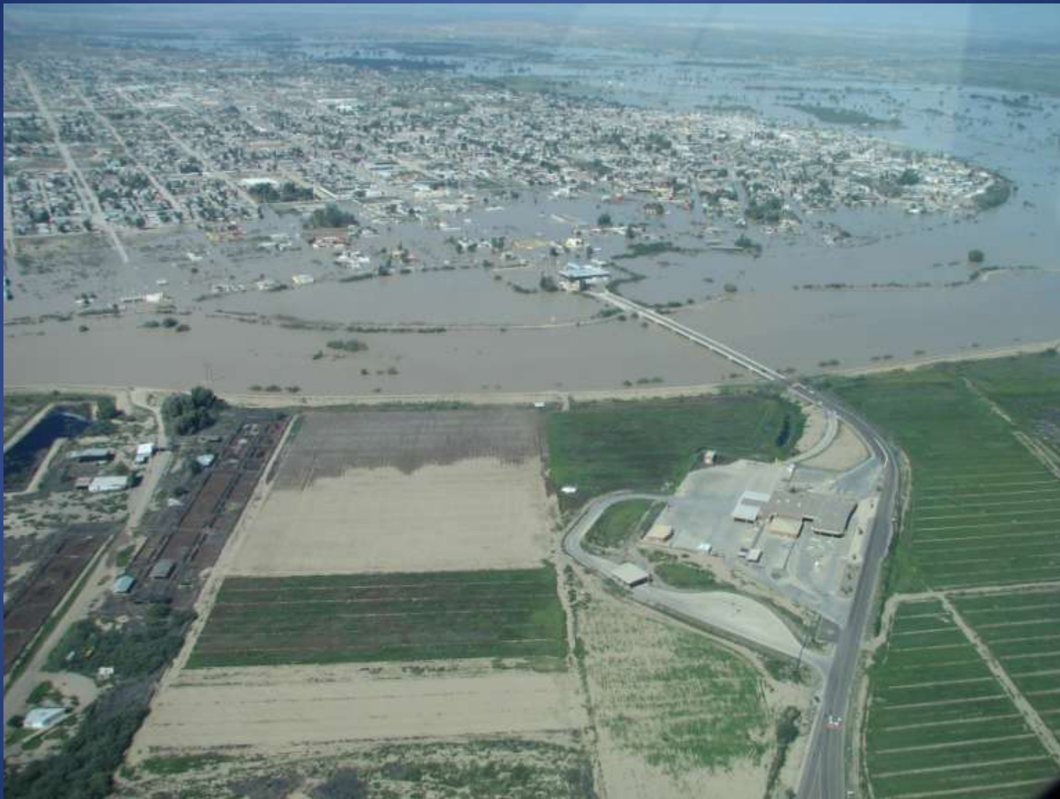
Rio Grande at International Bridge RG_09_20_08 054
