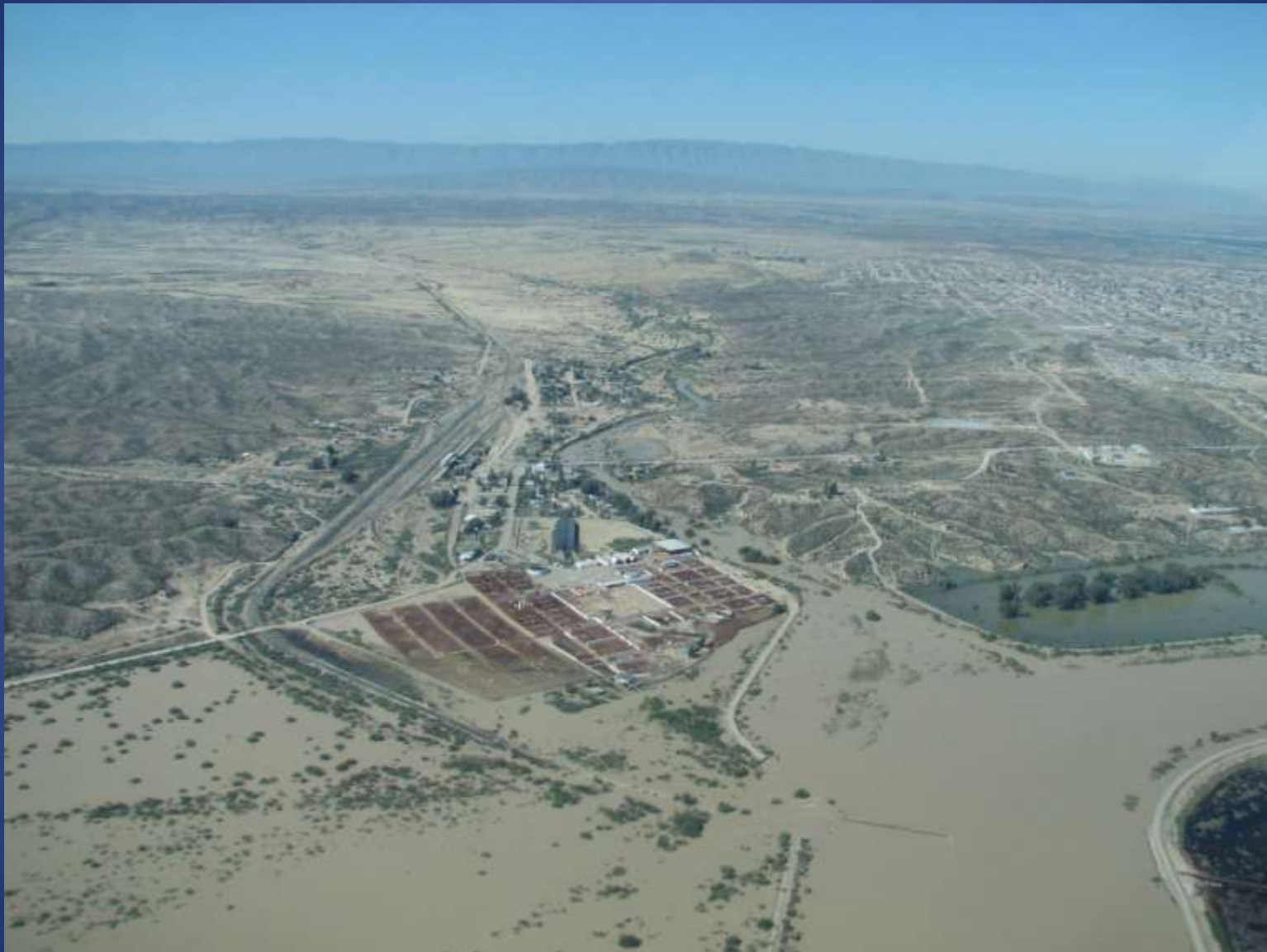
Rio Grande at railroad bridge crossing downstream of Presidio (MX in background).
