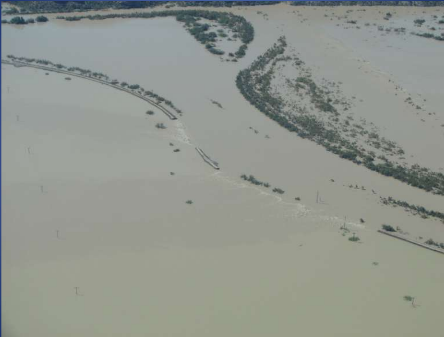
Closer view of previous picture. Overtopping levee downstream of Presidio golf course. RG_09_20_08 080
