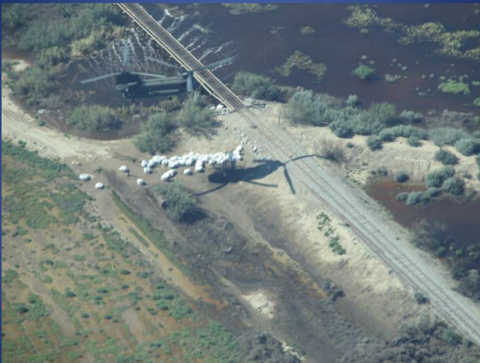
U.S. Army Chinook helicopter sandbagging along Railroad bridge crossing Rio Grande downstream of Presidio.
