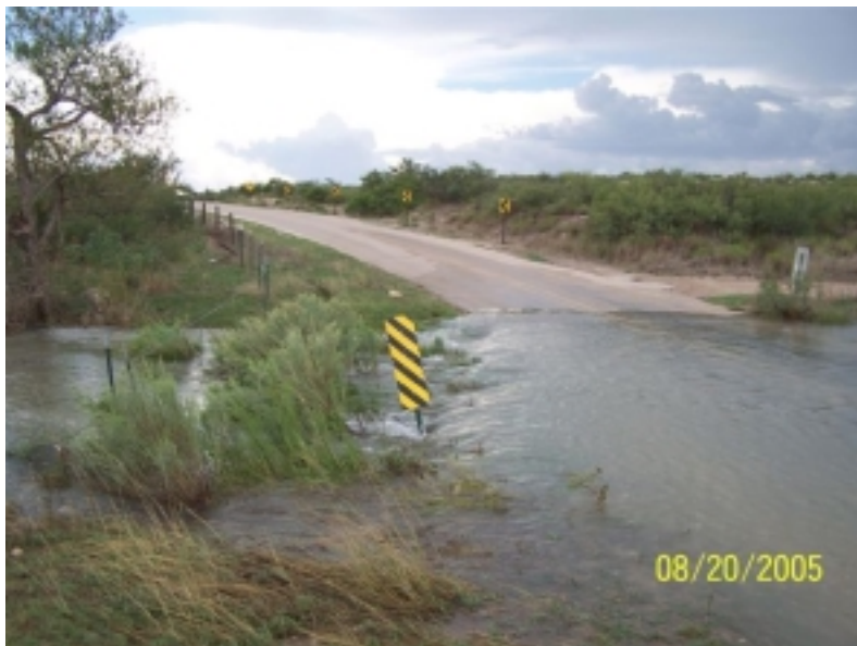
Flash flooding on Eddy County Road 720. The photographer reported that water depth was two feet. Photo Courtesy: Wendall Malone
