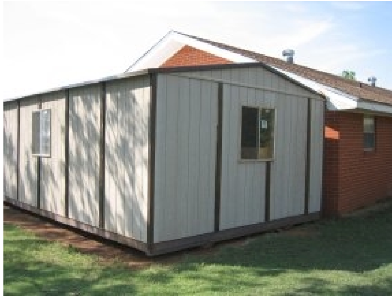
Looking closely at the picture, one can see that the shed has been moved about a foot and a half towards the house, stopping only after it hit the house. Photo courtesy: NWS Midland Damage Survey Team
