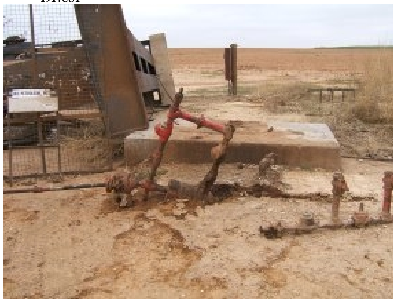
A pump jack was pulled out of the ground by a tornado in northwestern Martin County. Photo courtesy: Mark Cochran
