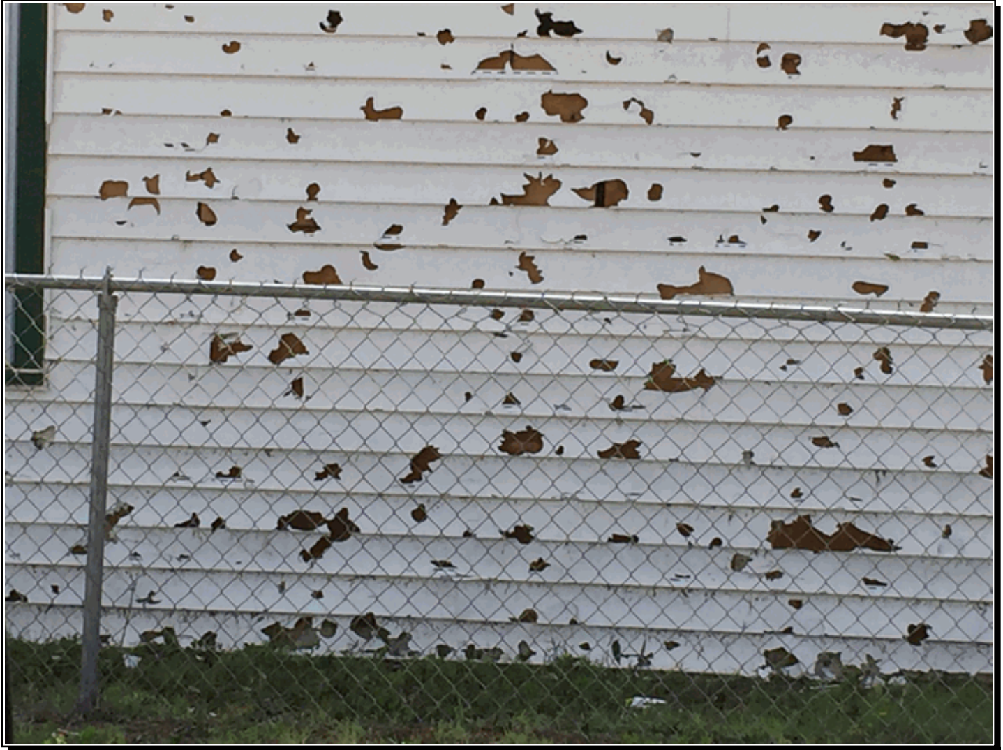
Tennis ball sized hail in Seminole, TX that stripped the siding off of houses. Photo courtesy of Mark Strobin.
