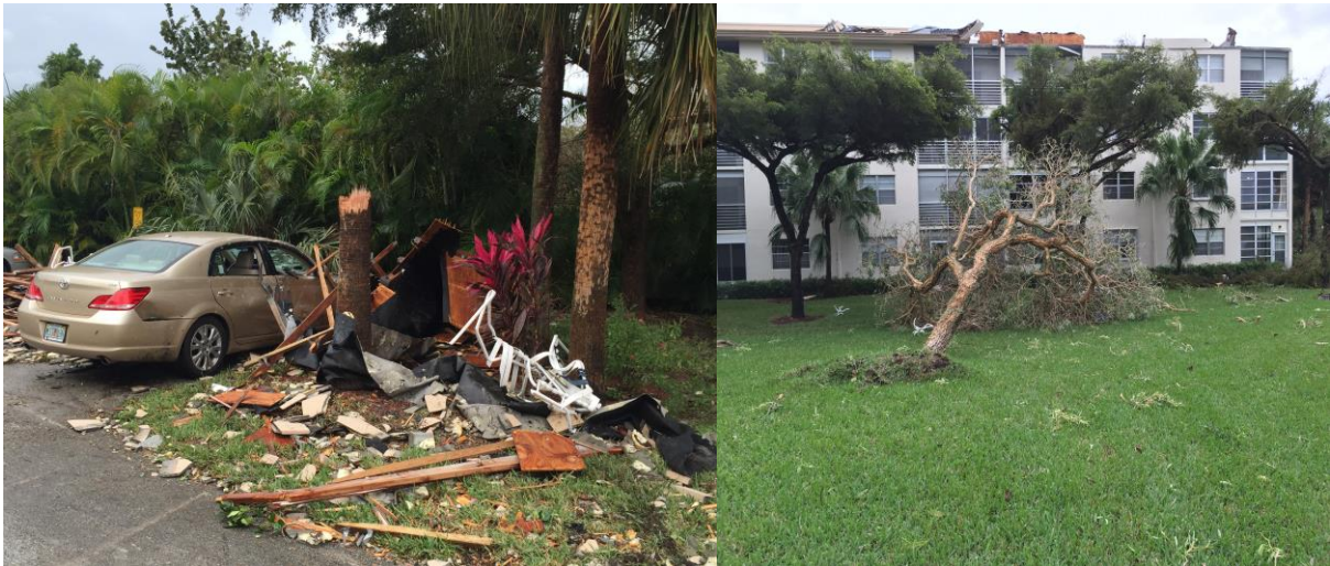
Tree and roof damage in Coconut Creek/Wynmoor Village
