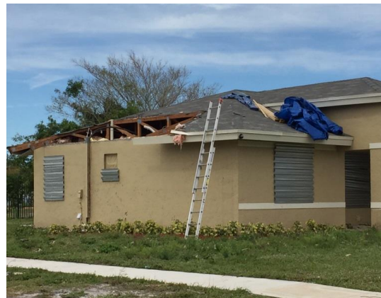
Pompano Beach Damage
