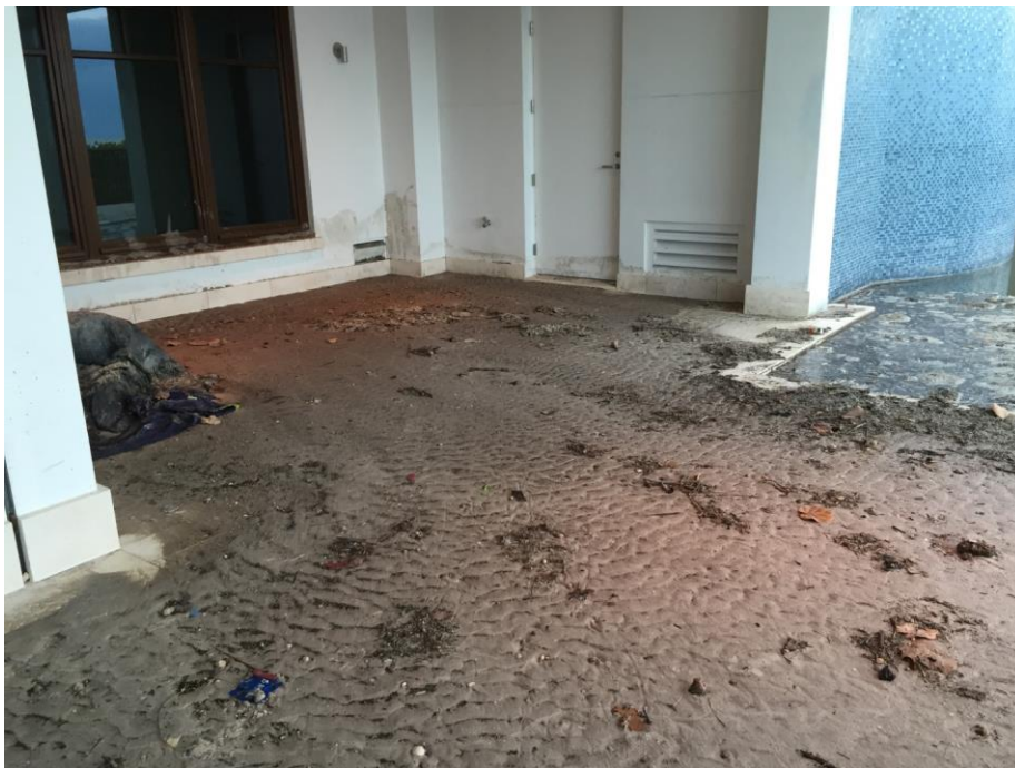
Beachfront home in Naples with water marks on building. Picture courtesy Jessie Settle
