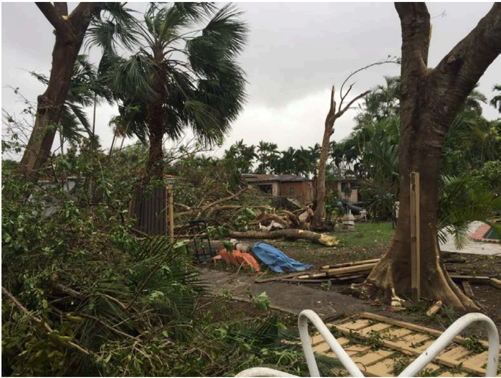
Trees and home damaged by tornado in Miami Springs on January 23 rd (NWS Storm Survey photo)
