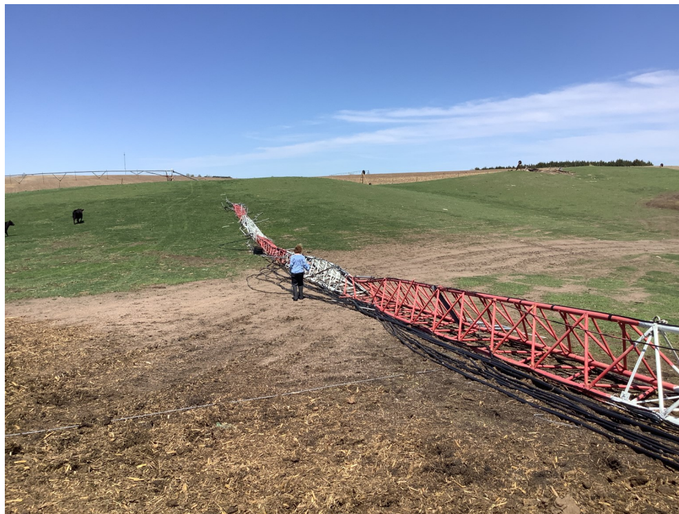
Figure 3. The 300 foot communication tower that collapsed near Hartington
