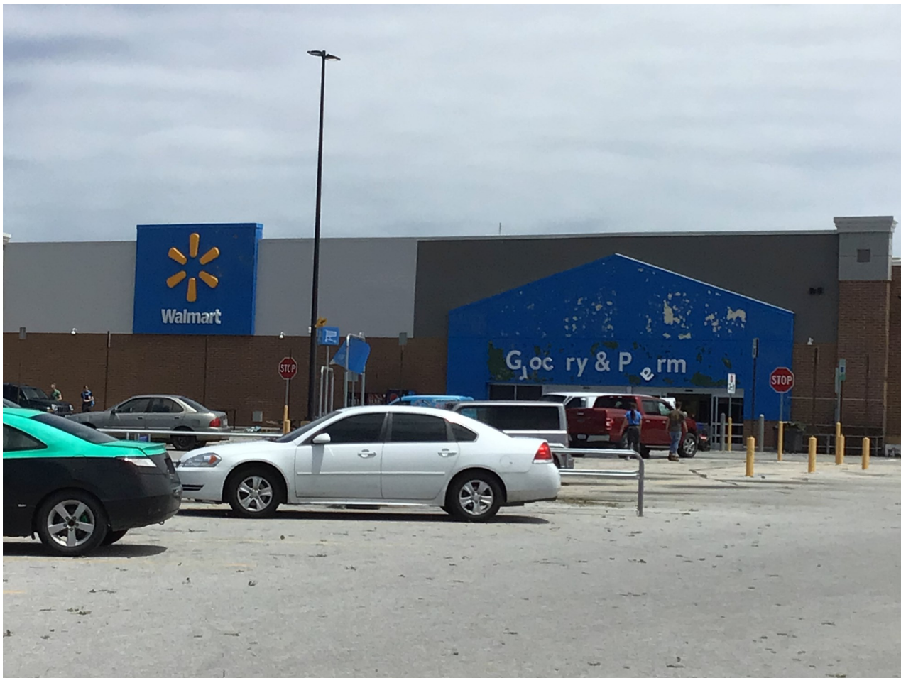
Wind-driven hail decimated the store front of the Wal-Mart on the south side of Seward. NWS photo.
