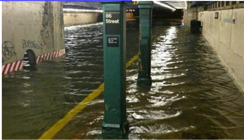
(Dumbo) 1-3 ft of inundation along East River in Dumbo neighborhood under the Manhattan Bridge
