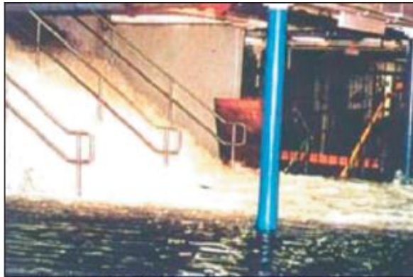
Flooded PATH Station - 1992 Nor'easter
