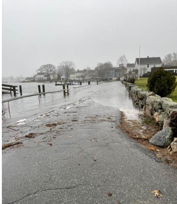
Groton End of Shore Avenue along Thames River inundated
