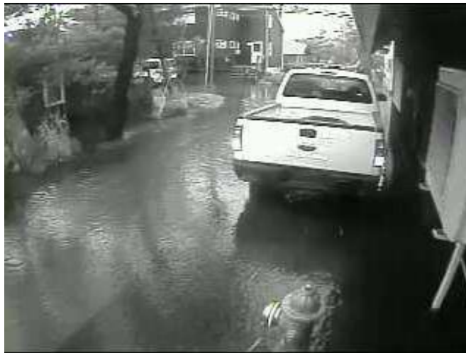
Inundation into Ocean Beach Firehouse . (1/24/2017)
