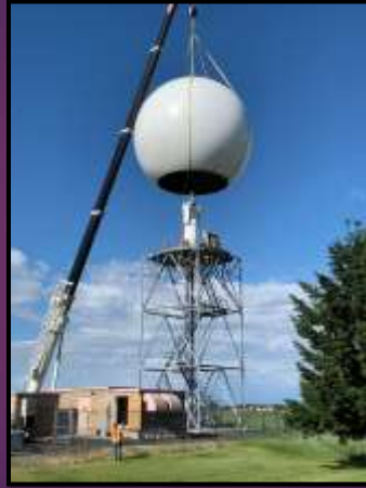
Installed in 1995 – Pedestal Replacement 2019
