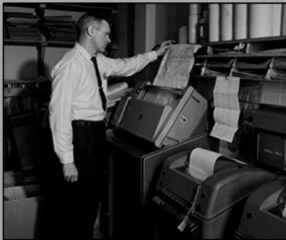
Facsimile machine that printed weather maps using wiper blades and electronic signals
