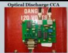
Stack Monitor CCA
