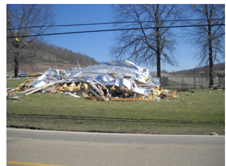
Damage from the EF-2 tornado off of Route 136 in Sewickley Township.
