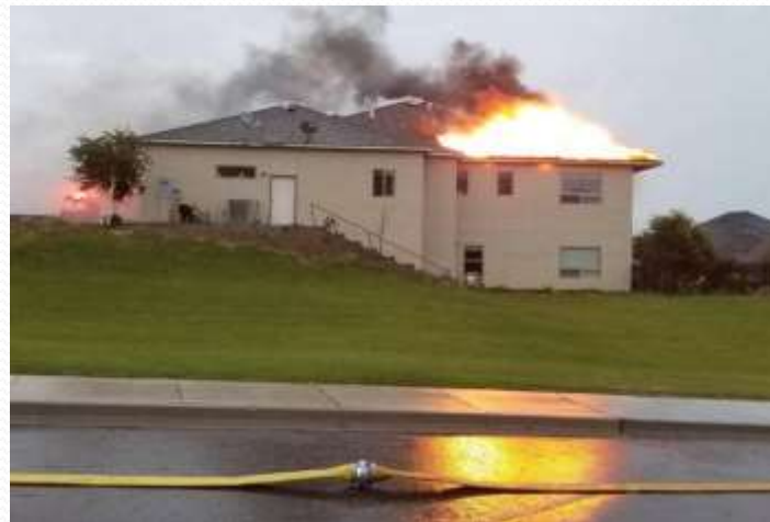
Lightning set fire to a house in the 1400 block of Meadow Hills Drive in Richland, WA on June 26 th as a severe storm moved through. Photo Courtesy: Rick Larson & Tri-City Herald
