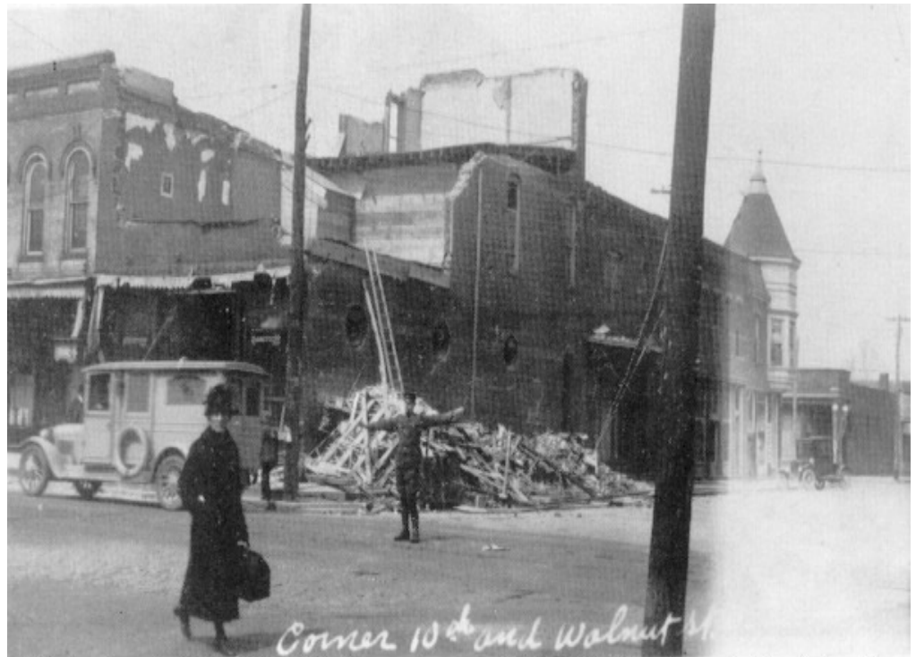
Originally a three-story building, Werner's Drug Store on the corner of 10th and Walnut Streets was reduced to only two stories. Photograph courtesy of the Jackson County Historical Society in Murphysboro, Illinois.
