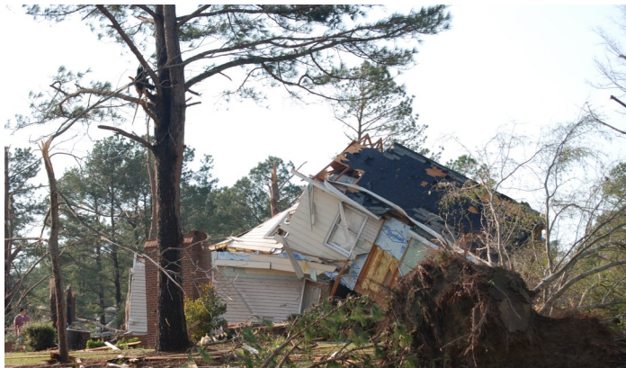
Tornado Damage from 2011 (NCDPS-NCEM)
