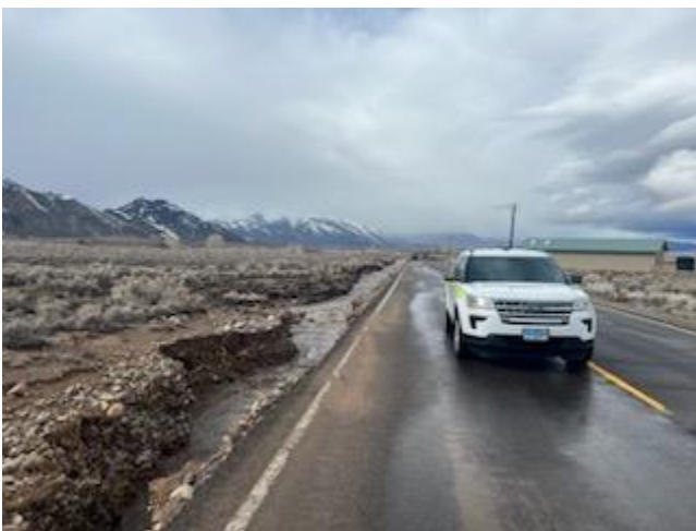
Figure 3. Eroded shoulders along NV-338. Photo credit: NDOT
