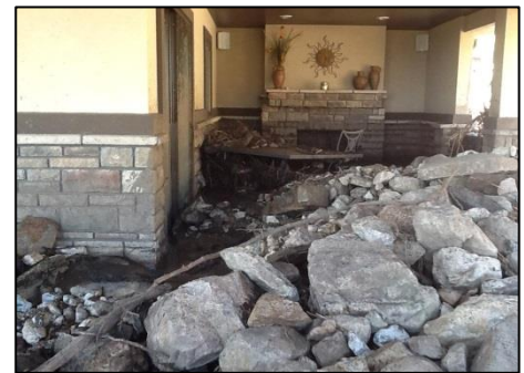
Fig. 3 – An intense thunderstorm caused flash flooding and debris flows downstream of the Sheepherder Hill burn scar
