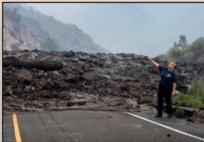
Figure 3) Debris flow on Highway 38 near the Valley Fire. Source: CalTrans District 9.
