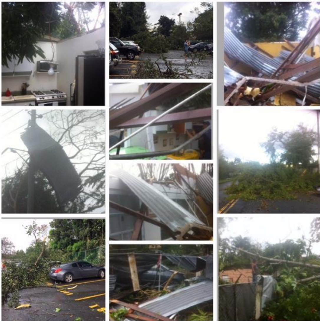
Figure 6: Damage associated with the strong winds at Villa Andalucia and Park Gardens, Rio Piedras.
