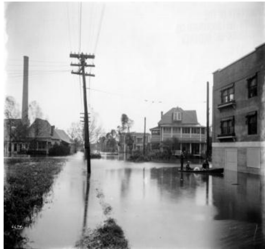
The storm surge brought extensive urban flooding as shown here at the intersection of Parker and Eagle streets, Tampa.*
