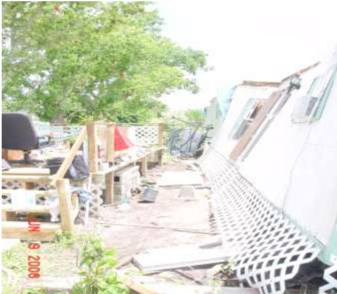
Un-anchored single-wide mobile home pushed 4 to 5 feet from original position. Mobile home roof was blown off and walls partially collapsed. Notice the almost intact trees to the west of the home. Several small 4 inch diameter branches were broken; however, trees remained mostly intact.
