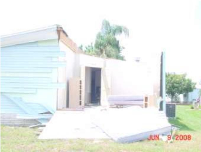
Double-wide mobile home with complete structural failure of outer wall and roof section. Wall joints were screwed together 2X4 sections with 2X4 pieces split vertically. Wood was not rotted.
