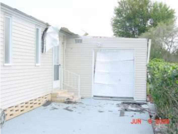
Roof damaged, but not removed from main double-wide trailer. Garage door blown in with garage roof blown off and thrown 100 yards. Items in the garage remained in their places during event.
