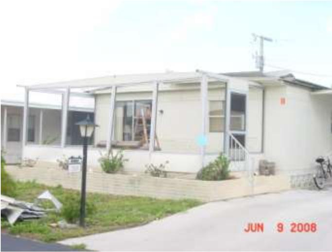
Double-wide mobile home with roof damage. Screened porch (lanai) severely damaged with roof missing as well as outer walls. Mobile home aluminum roof shredded in places.
