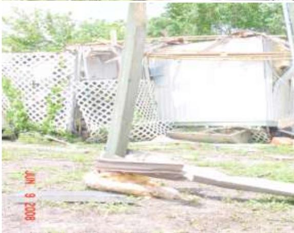
More roof and wall damage along with aluminum wrapped around a wooden pole. Bottom image is close up on aluminum roof with roofing nail visible. The roof was attached by evenly spaced nails with no other substantial reinforcement.
