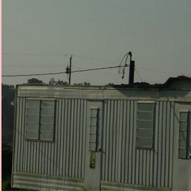
Mobile home damage: It doesn't take much! All of these were from F0 tornadoes. Leftmost photo: Roof damage, Wauchula, Hardee County, from August, 2003; Center photo: Roof and siding debris, Zolfo Springs, Hardee County, May 2003; Rightmost picture: Roof off of a mobile home in Citrus County, March, 2001.
