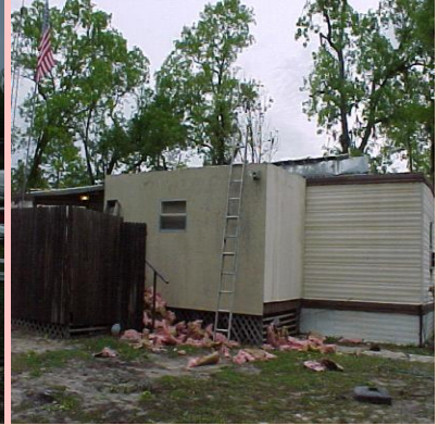
Mobile home damage: It doesn't take much! All of these were from F0 tornadoes. Leftmost photo: Roof damage, Wauchula, Hardee County, from August, 2003; Center photo: Roof and siding debris, Zolfo Springs, Hardee County, May 2003; Rightmost picture: Roof off of a mobile home in Citrus County, March, 2001.
