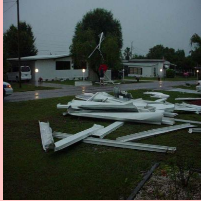
Mobile home damage: It doesn't take much! All of these were from F0 tornadoes. Leftmost photo: Roof damage, Wauchula, Hardee County, from August, 2003; Center photo: Roof and siding debris, Zolfo Springs, Hardee County, May 2003; Rightmost picture: Roof off of a mobile home in Citrus County, March, 2001.
