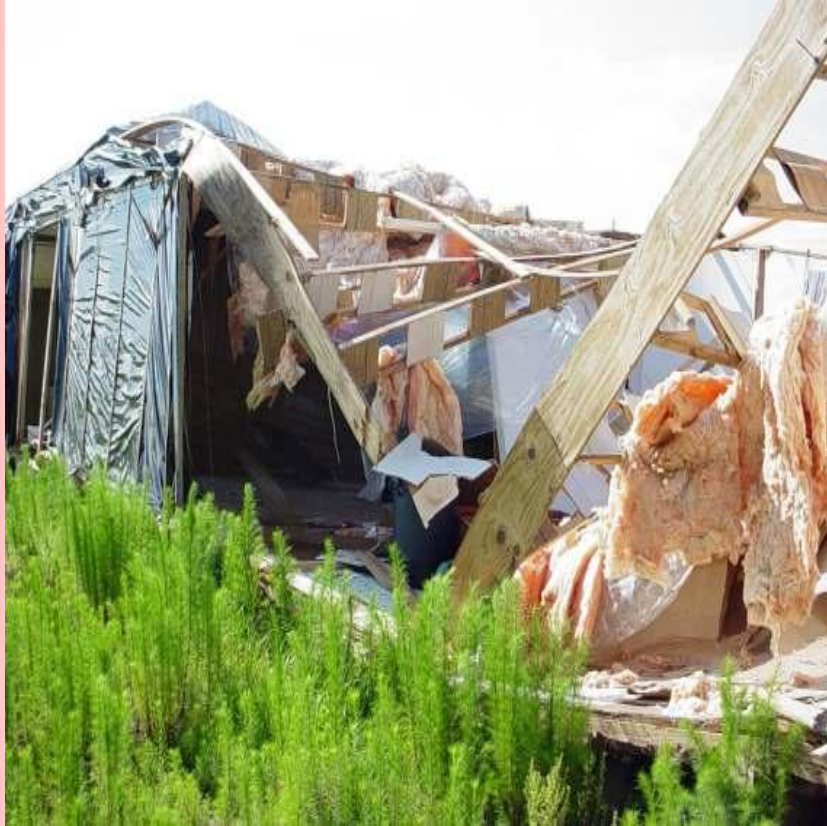
Destroyed mobile home in Hardee County. Photograph courtesy of Hardee County Emergency Management, 2003.
