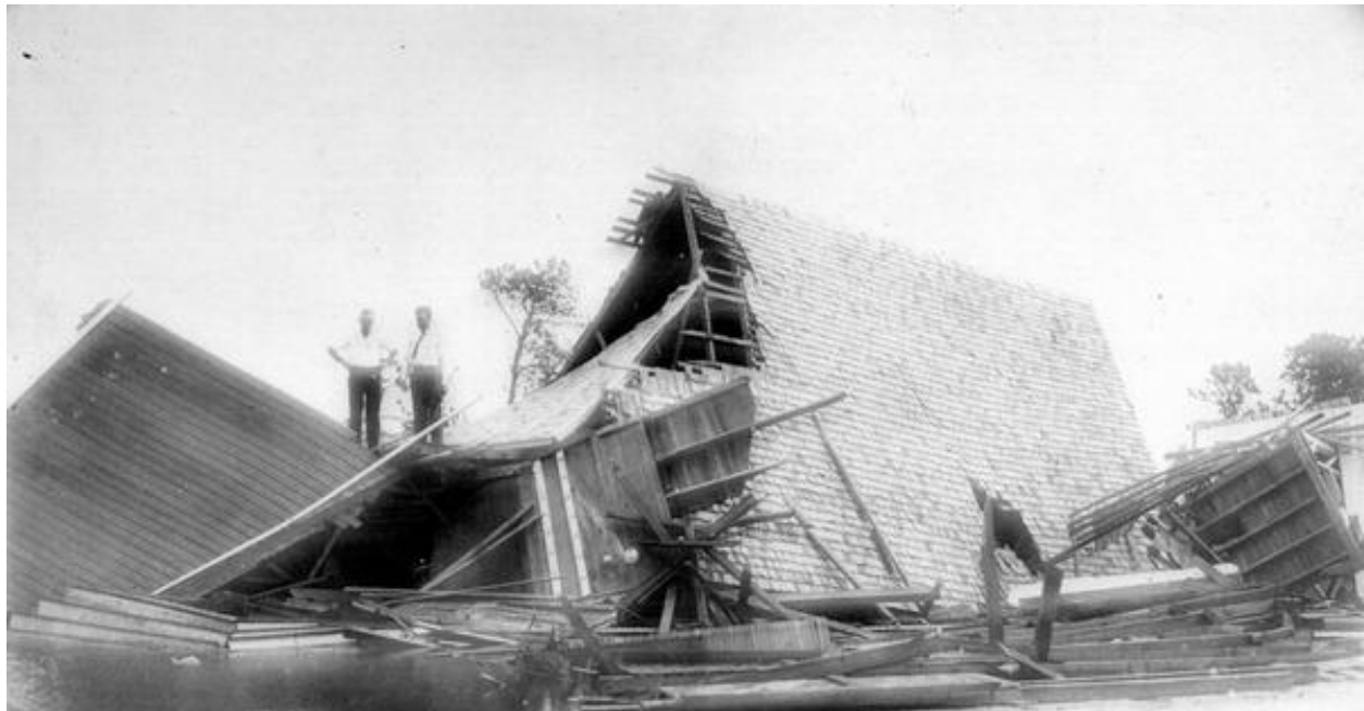
Figure 1. Damage to Knight's Chapel in Nokomis, FL
