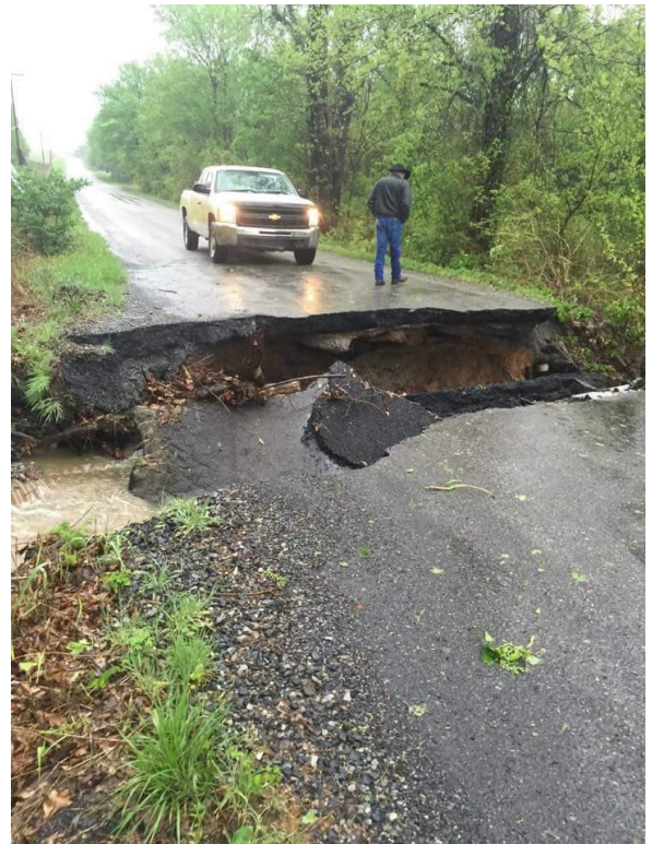
Fig 6. 4/13/2015 High Hill Rd. between Alderson Rd & Bache Rd near McAlester (via twitter @dljames0001)
