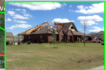
EF-1 damage to a home under construction (above), and a nearby completed home (below).
