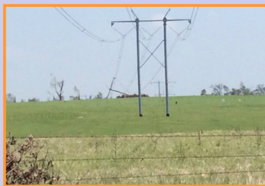
Above: A large metal transmission tower destroyed near Boswell, OK. This corresponds to EF-3 damage.
