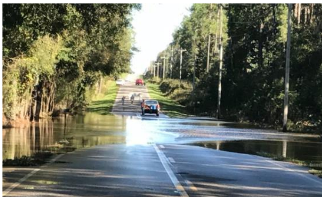
FIG. 7. Photo tweeted by Baldwin County EMA at 2030 UTC showing the low-water crossing point on County Road 48 near the Fish River Bridge.
