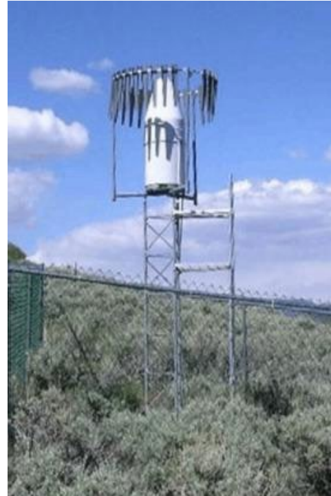
Figure A-3. Fischer-Porter Gauge on a Snow Tower with Wind Shield.
