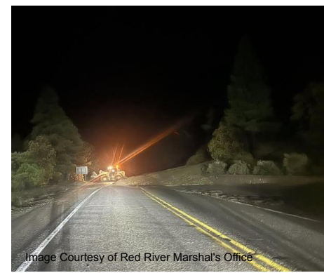
Mudslide on NM Road 38 - Oct 16th
