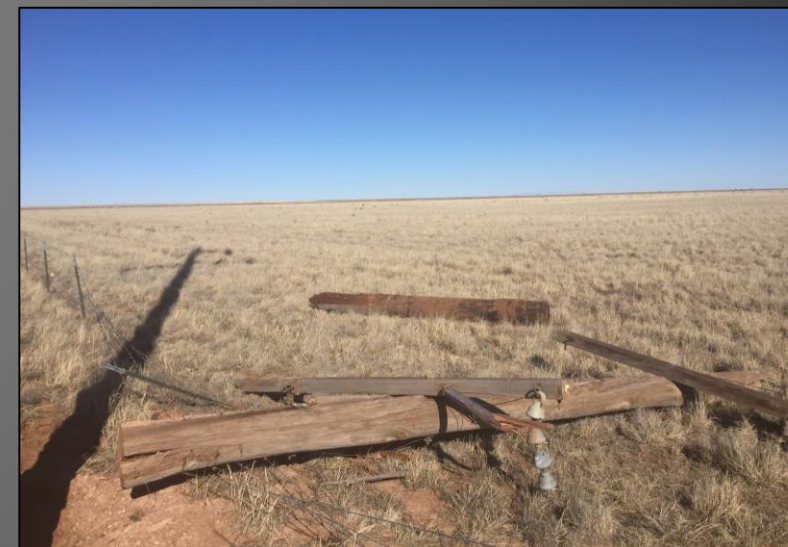
Broken power pole. Photo by NWS Albuquerque.
