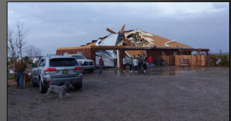
Damage to a home in Dexter. Photo by Jim Tucker.
