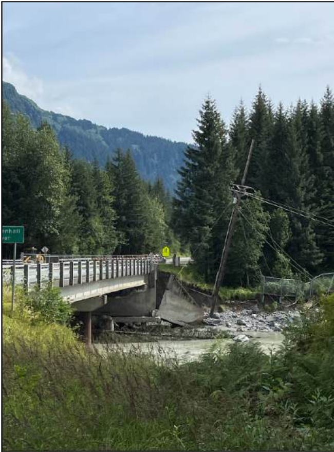
Image 1: Damage to Back Loop Road Bridge and a telecommunication/power pole. Photo courtesy of NWS.
