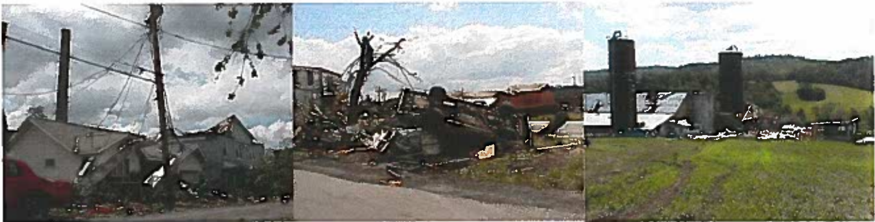
Photos of damage in Mechanicville and Stillwater, New York, except picture in lower right from Hoosick, New York.
