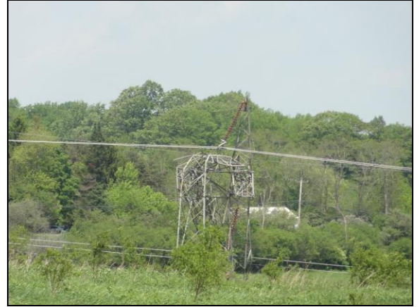
Figure 3: A high-tension power line tower destroyed (one of five severely damaged along this stretch). This was seen from NY Route 159 and North Kelly Road.
