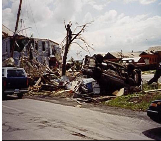
Figure 5: F3 damage from the Mechanicville Tornado of May 31, 1998 (NWS at Albany photograph).
