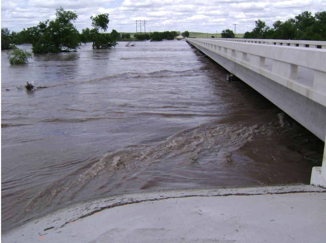
**Wolf Creek at the Texas State highway 305 bridge at Lipscomb. Looking north along the upstream side of the bridge. Note the high water mark on the bridge abutment.**
