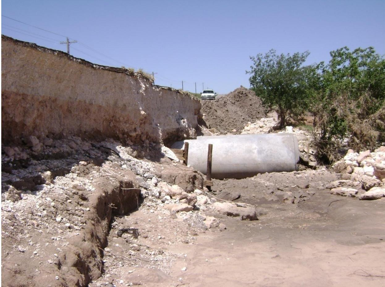
**Water washed out the downstream side of F.M. road 759 at the south fork of the Wolf Creek, 3 miles east of State Highway 70.**
