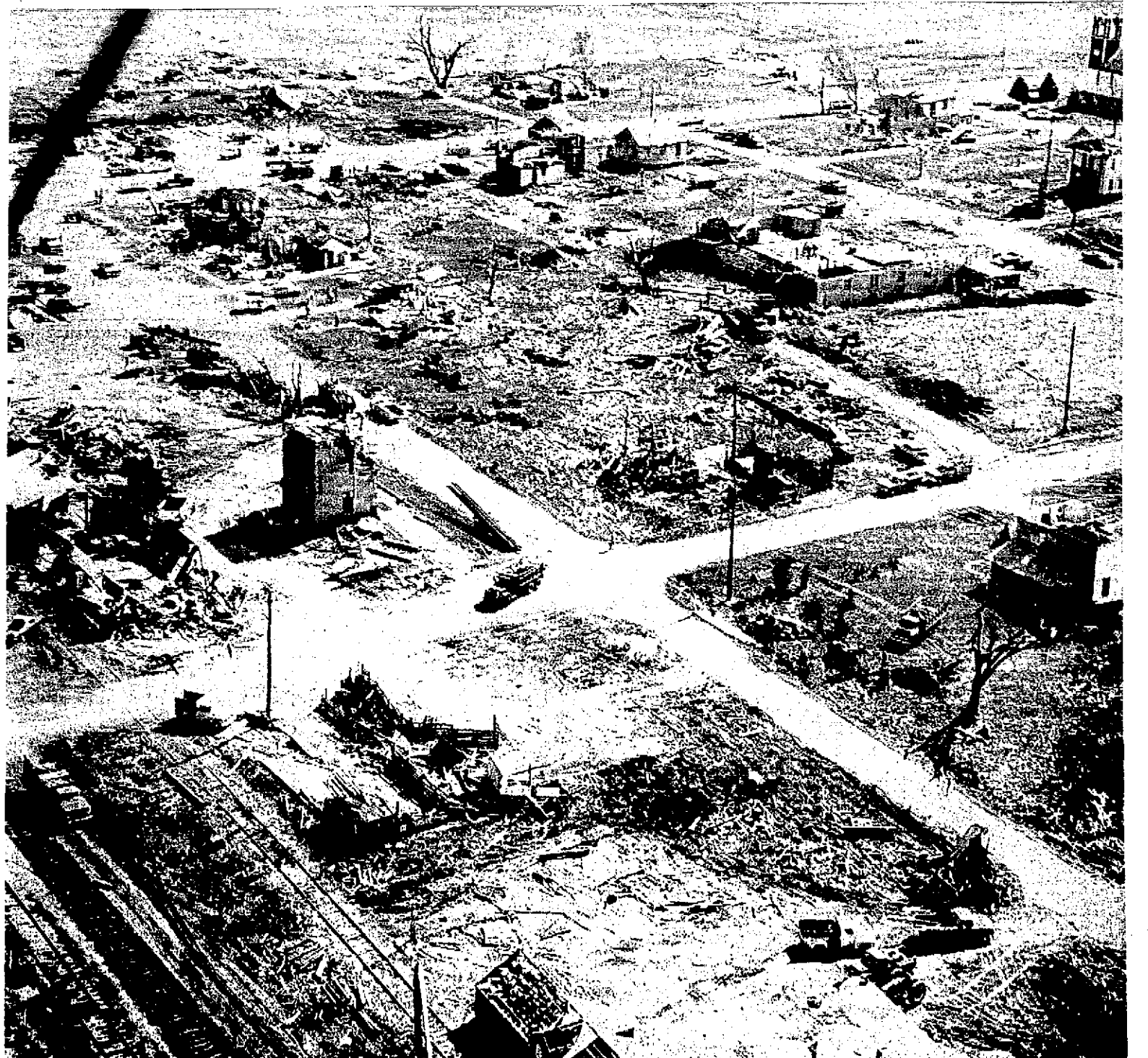
MAYNARD DEMOLISHED —The town of Maynard was, proportionately, as demolished as Oelwein or Charles City Wednesday, May 15, when the twin twister struck northeast Iowa and left in its path 18 residents dead and over $35-million in real estate lost. In the above photo the twin twister struck northeast Iowa and left in its path 18 residents dead and over $35-million in real estate lost. In the above photo shot by City Editor Earl Davis through the use of a National Guard helicopter, Iowa 150 runs along the top of the photo. At right the old St. Paul's Lutheran church bell tower remains standing, but just to the left the wall with windows is what remains of the new St. Paul's set to hold its first service Sunday. All business (top) across Iowa 150 were demolished, as well (lower left) as the cattle yards and Maynard Coop. The structure at lower right is what is left of a line of homes destroyed toward the north, including homes of Glenda Kelly, 3, and Mrs. Louis Ponsar who died in the devastation.
