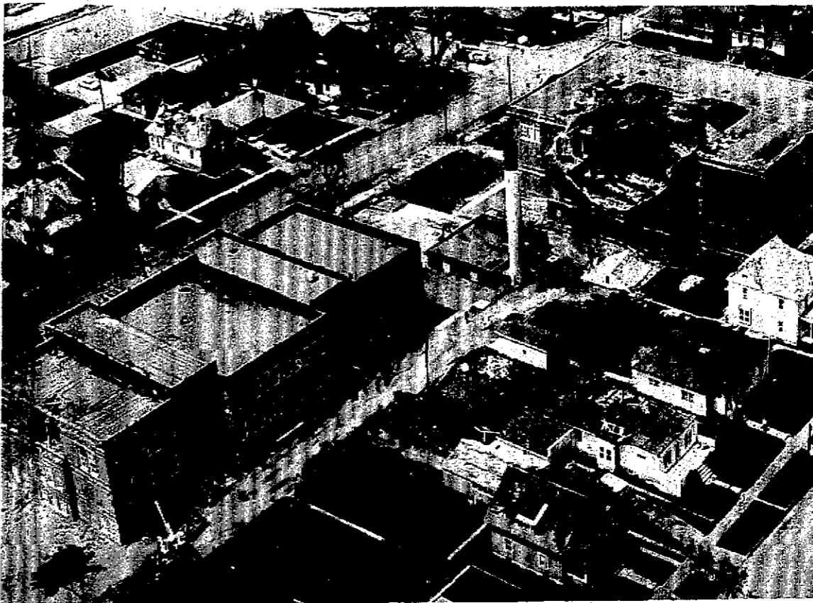
SCHOOL DAMAGE—The Oelwein Junior High building (upper right) suffered extensive damage. The Junior High roof was ripped off the building and a gaping hole remains in the structure. The Central Grace School (lower left) suffered heavy roof and structural damage.
