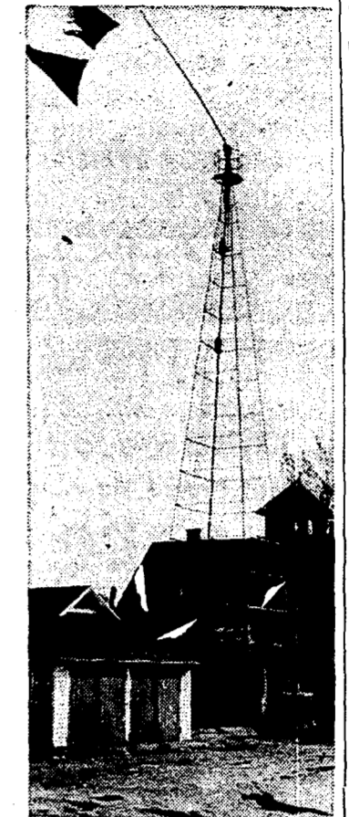
Even the storm warning signal tower at the coast guard station was not exempted from the storm. The staff at the top of the tower was bent at a 45 degree angle by the heavy wind.
