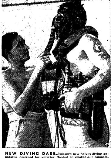
Air in bag is regulated by valves on the weighted belt.
