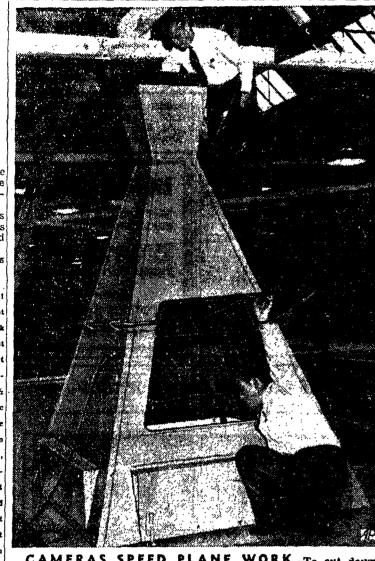
CAMERAS SPEED PLANE WORK\_To cut down time interval between engineering on a new model plane and its initial flight two glant cameras are used in the Lockheed aircraft plant at Burbank, Cal. They make patterns for sections and parts under a new photo-loft-template process. Camera stands 10 feet high, uses a 19-inch focal length lens and plates half a yard long.
